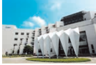
Tainan Plant (Diamond-rated Green Building)
