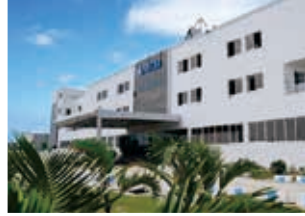
Rudrapur Plant (Green Building)
