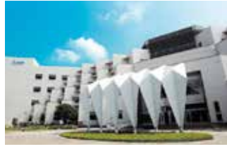
Tainan Plant (Diamond-rated Green Building)
